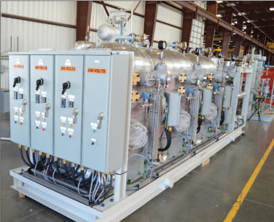
Multi-zone hot water for Sakhalin Island, Russia
