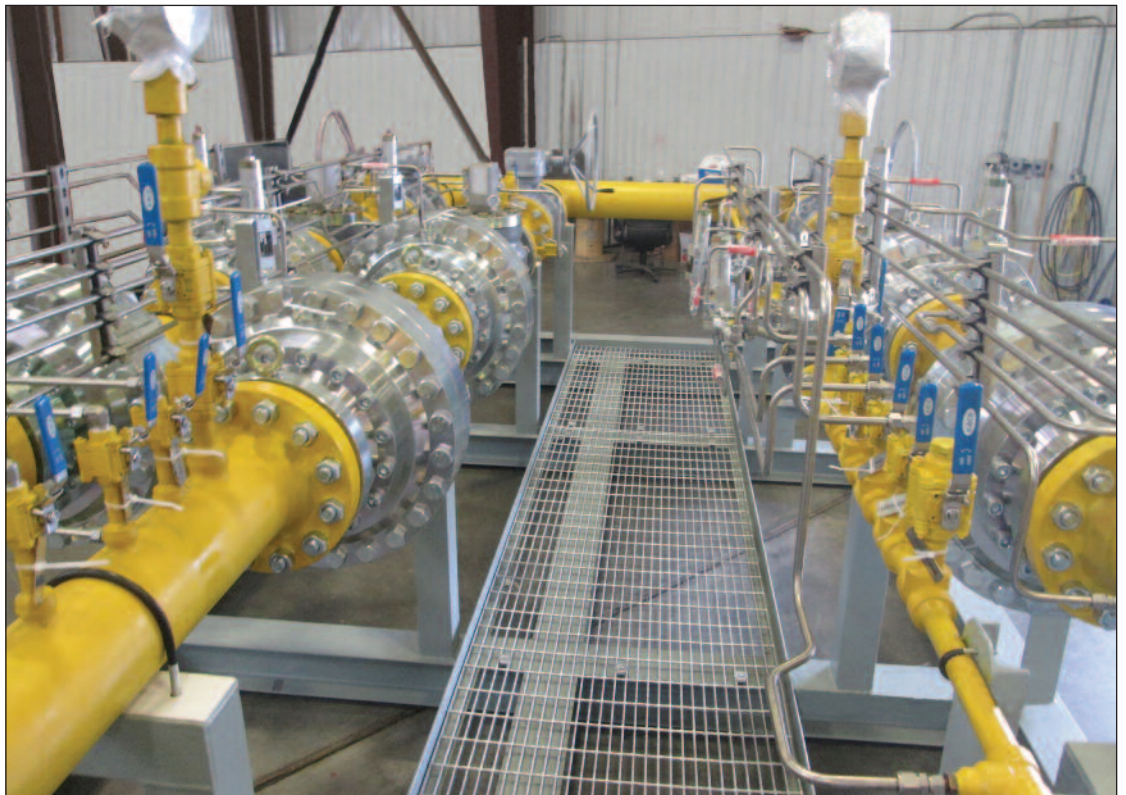
Wide-open monitor PCV arrangement
